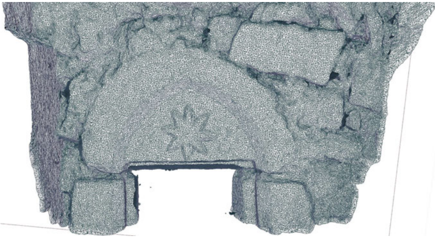
Fig. 21.6 An example of a high-LoD relict element, a photogrammetric model of a surviving door in the Criechinger Haus
