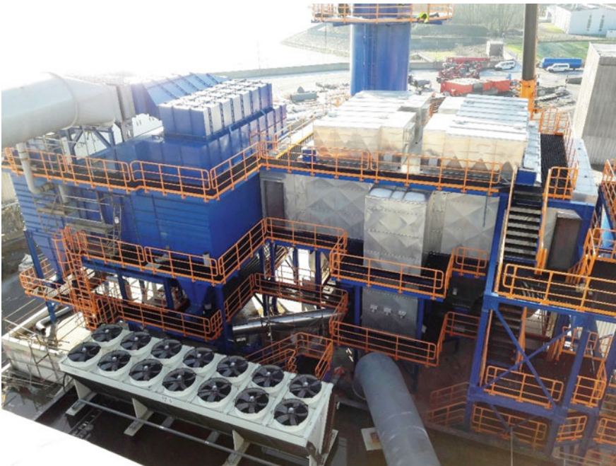
Fig. 3 Hygiene gas filter (left) and process gas filter (right)
