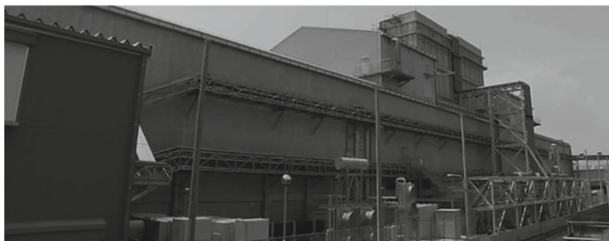
Fig. 4 The new No. 3 electrowinning plant
