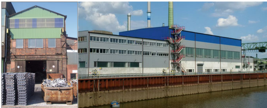
Fig. 2 Left: Old lead refining facility; Right: New lead refining capacity with offices for site administration
