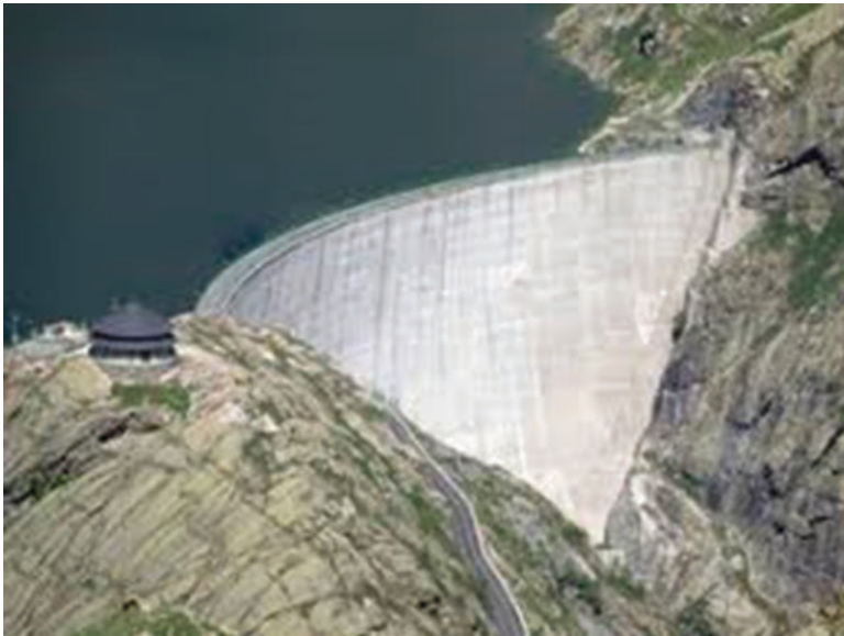
Fig 7.6 The Chiotas arch-gravity dam in Piedmont, 88 m tall, is a part of the Entracque hydro-power plant, actually the largest in Italy with 1318 MW installed (Source: ENEL 2012)
