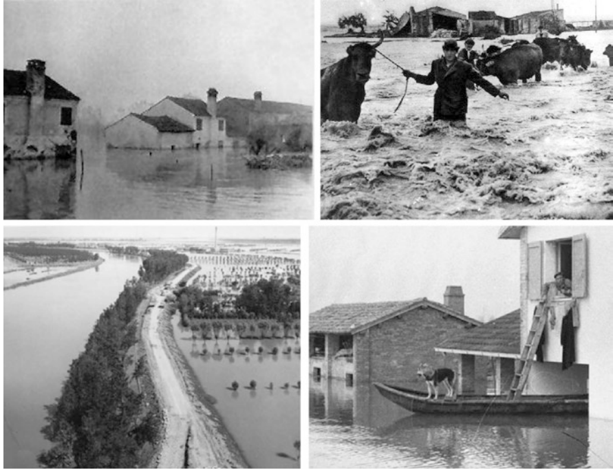
Fig. 11.3 Views of the Po River flooding in November 1951
