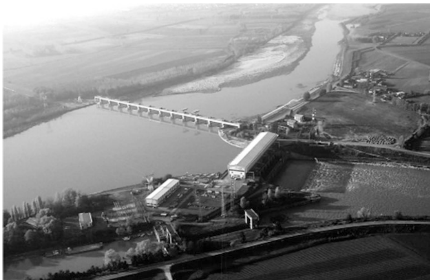
Fig. 7.7 The Isola Serafini power plant on River Po, with four 300 m 3 /s generation groups, is one of the largest run-of-river plants in Europe (Source: Bizzi et al. 2015)
