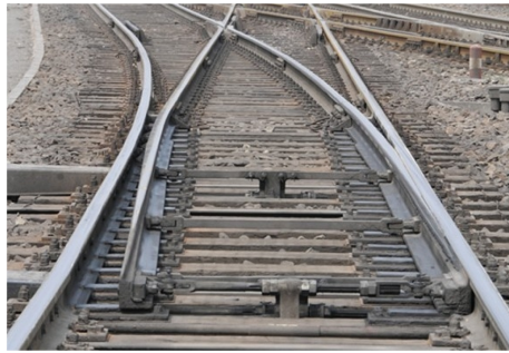
(b) Cross-high-speed railway turnout structure
