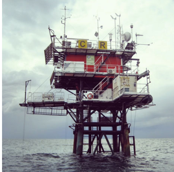
Fig. 5.2 The ISMAR oceanographic tower “Acqua Alta”, located in the Northern Adriatic Sea, 15 km offshore the Venice lagoon
