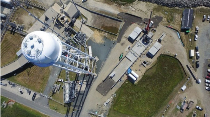
Fig. 14 Launch Complex 2 under construction in September 2019. (Graphic courtesy of Rocket Lab)
