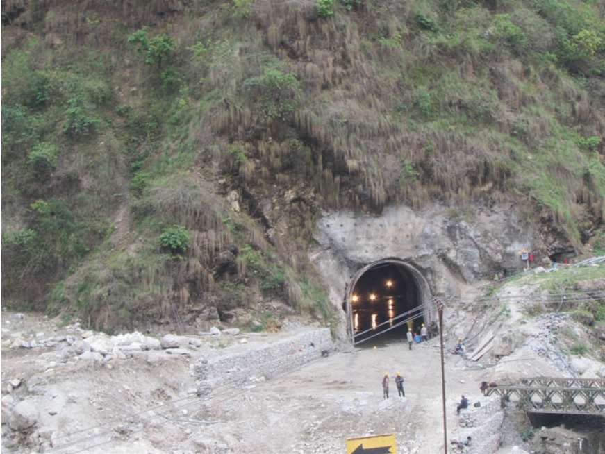
Fig. 30.3 A tunnel might make mountain gods pretty angry. (Photo credit: author)
