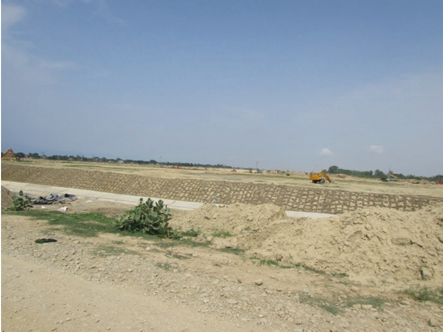
Fig. 4.4 Watershed modification in wetland regions, also done to protect against floods (earth works in a wetland area the new airport at Lumbini, Nepal, is shown here!
