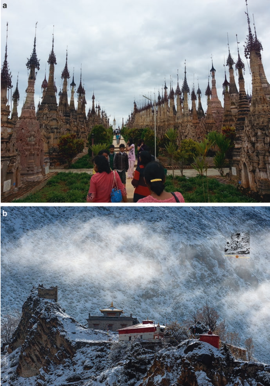
Fig. 14.7 (a) A high concentration of temples and monasteries in Myanmar. (b) A high pass temple (Credit: WWW and T. Ghale)
