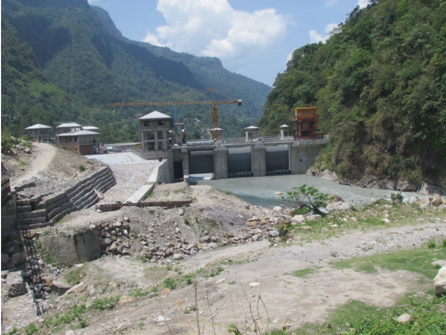
Fig. 31.1 Photo of a typical barrage section of a river in Nepal. (Photo credit author)
