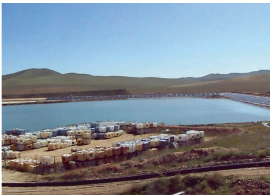
Fig. 41.6 Tailings storage facility of Boroo gold. (Photo: Rajive Ganguli)
