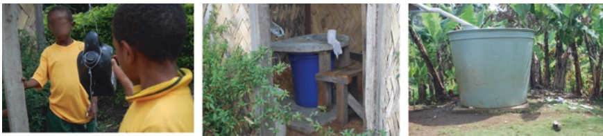
Fig. 9 WASH infrastructure installed by the Madan Water and Sanitation Project. Tippy taps for handwashing, a toilet built on the idea of reusing human waste for agricultural purposes and water catchment tanks (empty May–August in the dry season and surrounded by trash at the time of the photo) provided some infrastructure for WASH practices at four village schools. These photos were captured as part of the user research activity of observing schools. (a) Warike Elementary School children interacting and using Tippy Taps installed for handwashing. This is an alternative to the rain catchment tanks during the dry months from May to August; (b) To address the lack of running water composting toilets were installed in some schools. After bowel movements sawdust is added to the waste converting it to compost; (c) A rain water catchment tank is a secondary source of water (primary: river) that has been installed in every school. During the dry months of May through August this tank is empty therefore teachers and students have to walk to Wagi river for water
