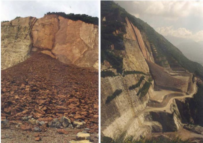
Fig. 17.21 Alpetto high rock cut slope (Cesana Brianza, Lecco, Italy) after the 1997 rock slide (Barla et al. 2012)
