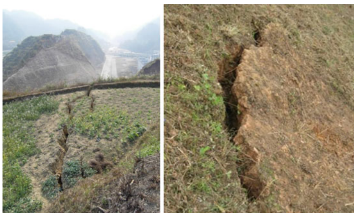
Fig. 17.8 In-site observation of surface cracks at the top of a slope
