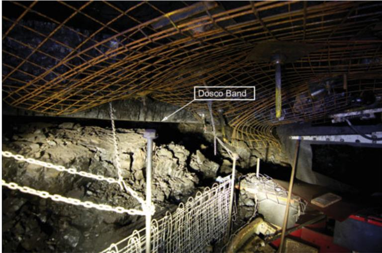
**Fig. 11.2** A coal burst event at Austar Mine, Australia. The coal rib burst out during roadway development. The overburden depth was 550 m. (After NSW Mine Safety Investigation Unit 2015)
