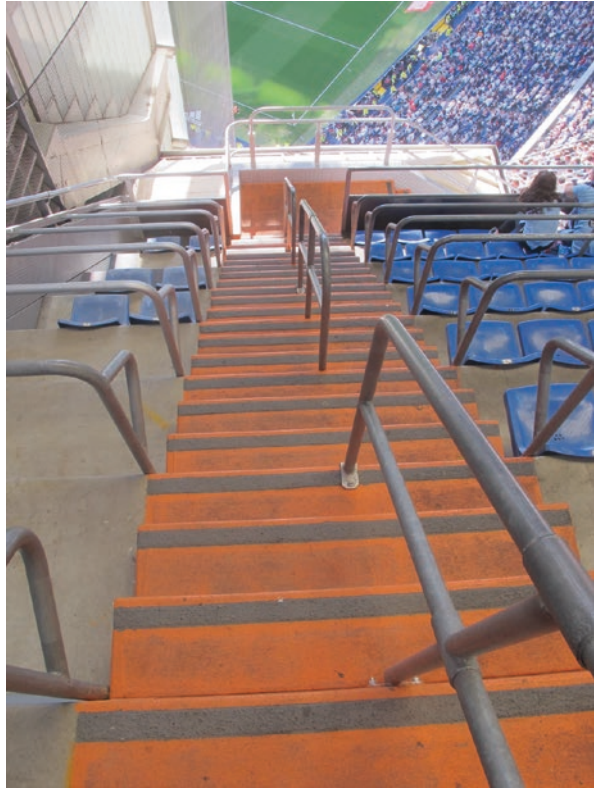
Fig. 28.3 Stairs and other architectural barriers in the upper deck of a large football stadium
