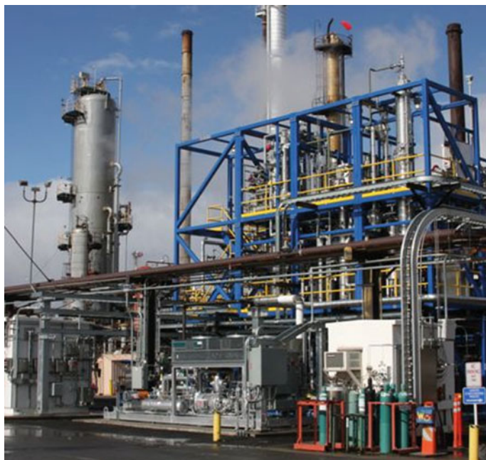
Fig. 2.1 ISOALKY Demonstration Plant in a refinery that consists of demo plant skids, cooling unit, and analytical shed (HF plant columns are shown in the background)
