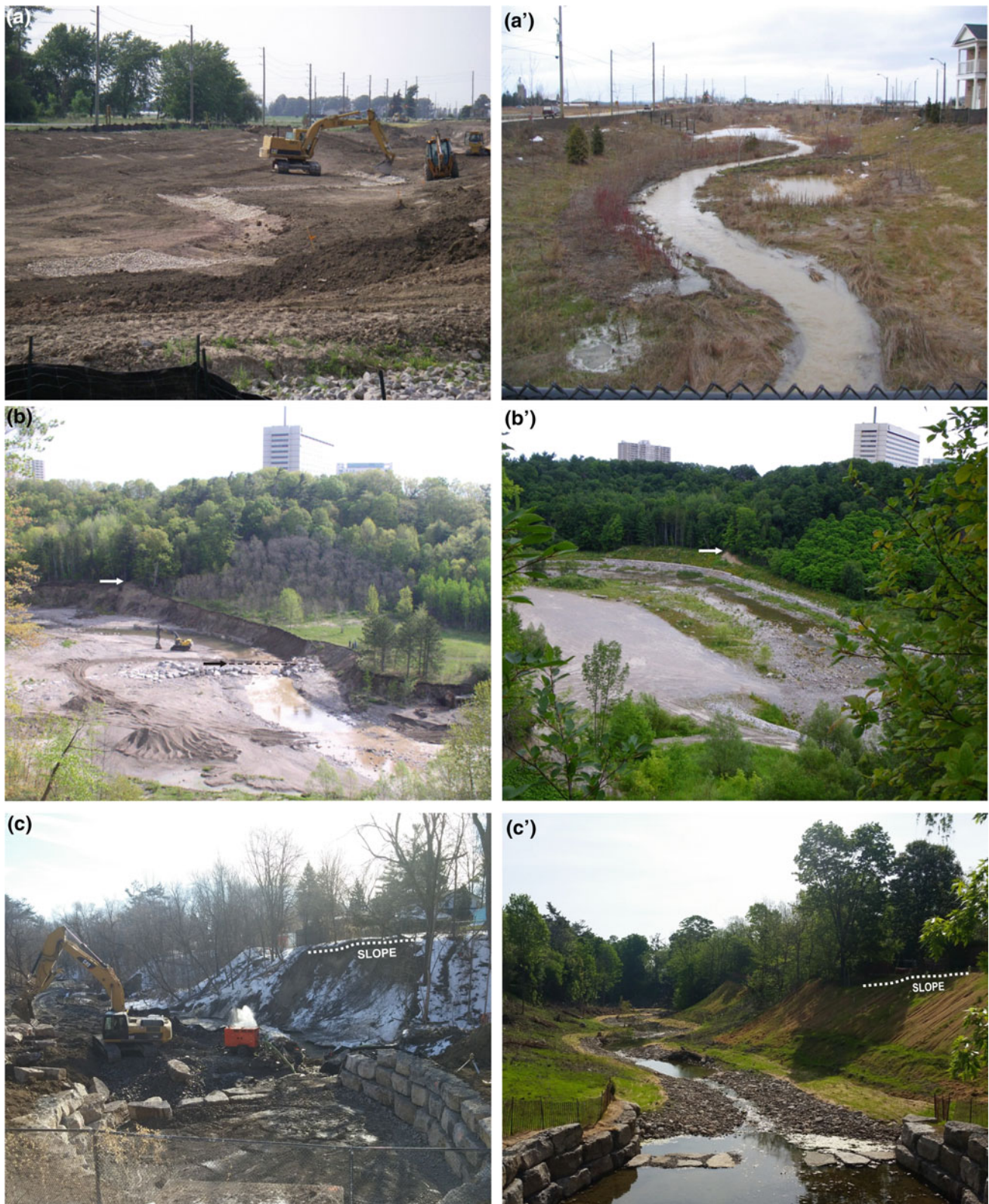
Fig. 11.13 Stream restoration and river engineering (before and after photos); a–a' stream restoration within formerly agricultural lands in the headwaters of Fletcher's Creek, Brampton a tributary to Credit River (see 4 in Fig. 11.1); b–b' river engineering to protect sanitary sewer pipe within Highland Creek (see 2b in Fig. 11.1), Toronto (white arrows for common reference point; black arrow and dashed line indicate exposed trunk sewer pipe in before photo); c–c' slope restoration and channel realignment within Amberlea Creek, Pickering
