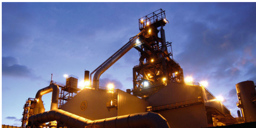
Fig. 2 Tata Steel Port Talbot, UK. Although not commercialized anymore, ammonia traces from COG processing can potentially be used for new purposes. Courtesy of Tata Steel, UK
