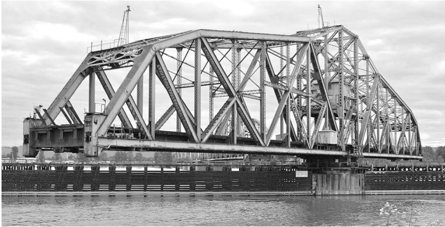
Figure 1. An open BNSF railroad swing bridge [18].
