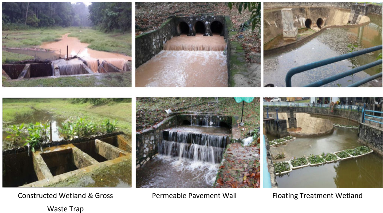
Fig. 5 Comparison of Alur Ilmu before (top) and after (bottom) implementation of structural approach (Mahmud et al. 2017b, c, 2018)
