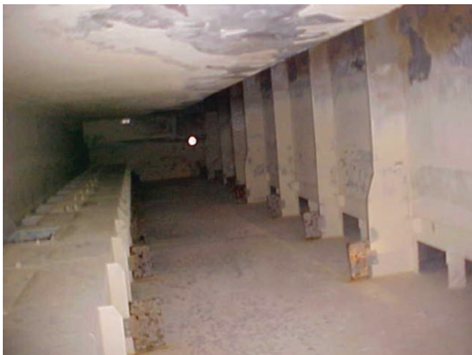
Fig. 5.8 Calcareous deposit covering most of the 1st stage flash chamber in MSF desalination plant
