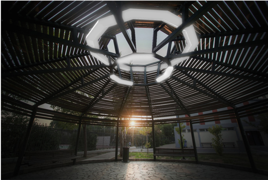
Fig. 3. View of the light and sound installation at the Serafio pavillion
