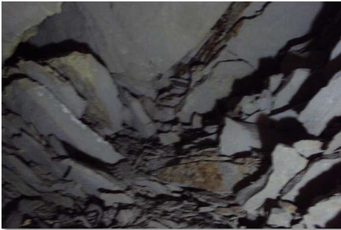
Fig. 9. Separation and failure of roof formation in galleries
