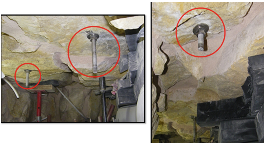
Fig. 13. Steel anchors to support shaft failure zone
