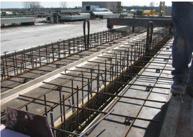
Fig. 3. BDT girders prior to concrete placement
