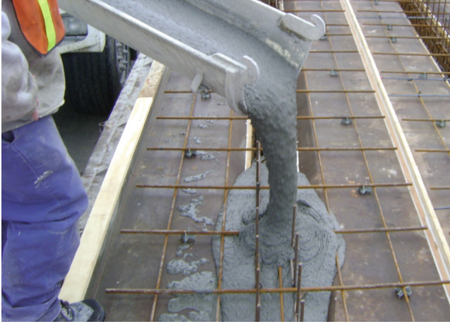
Fig. 4. HSSCC placed in double tee form
