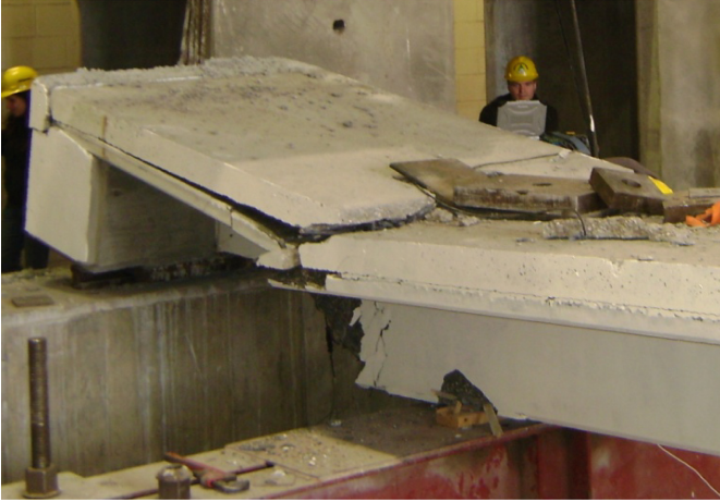
Fig. 15. BDT2 horizontal shear failure
