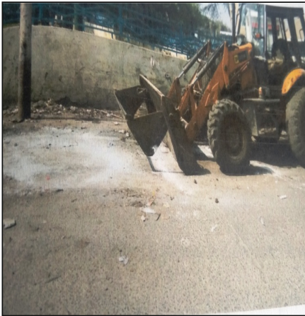
Fig. 8. Shows MSW spillage on the road (Bara Dwari).
