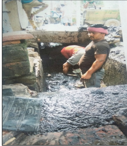
Fig. 3. Shows cleaning drains at Goolar road, Aligarh.
