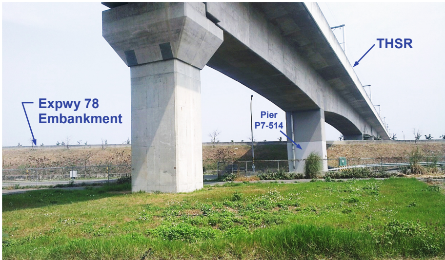
Fig. 5. Expyw 78 embankment and THSR piers and viaducts of the site (facing north)
