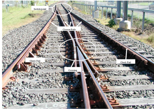
Fig. 1. Typical turnout geometry [7].
