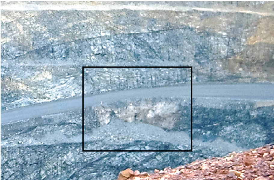
Fig. 4. Side-ramp failure (slabbing) at the open pit ramp, photo taken from the south in Feb. 2011
