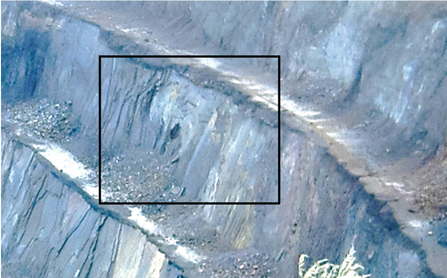
Fig. 3. Sidewall spalling in the face of the pit bench, photo taken from the south in February 2011
