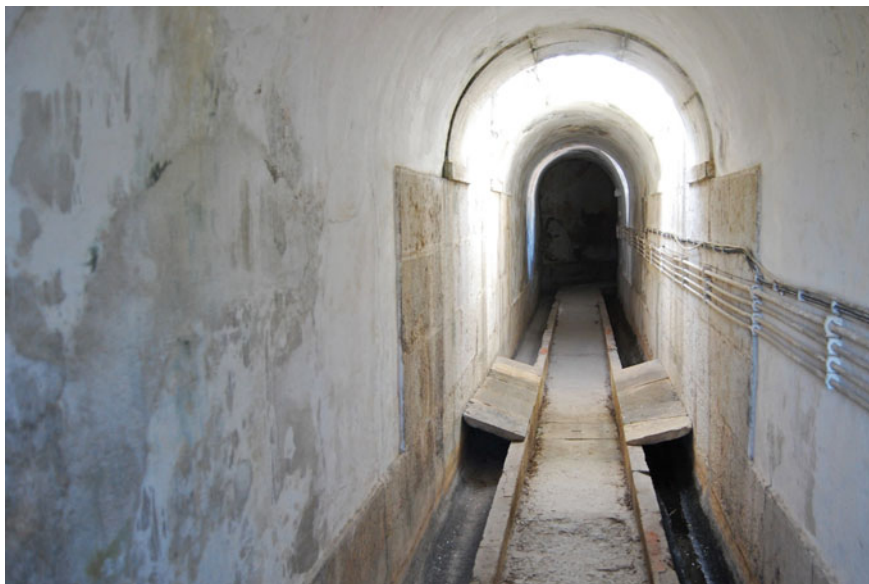
Fig. 3 Main aqueduct gallery depicting the water circulation gutters on each side of the central walkway. Photo courtesy of Pedro Inácio, 2010
