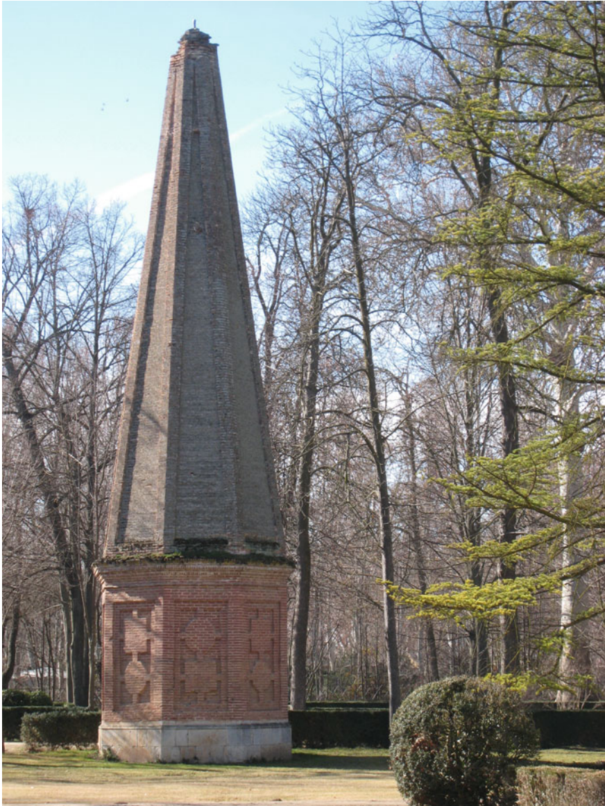
Fig. 8 Aranjuez (Spain) Jardín de la Isla, Irrigation Channel's Vent.; photo M. Merlos
