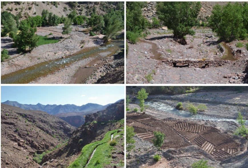
Fig. 8 The traditional irrigation system: little dams, channels, and ditches
