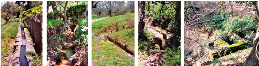
Fig. 6 Channels bringing water from the highest reservoir to the orchard near the house and other areas of the ensemble in La Fresneda. The last picture depicts the ruins of the water filter. Photos by the author
