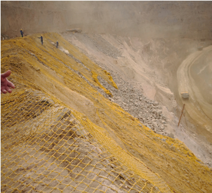
Fig. 3. Installation of high wall synthetic safety nets
