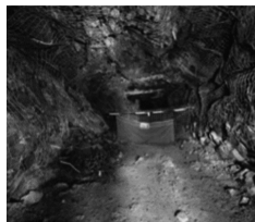
Fig. 1. Collapse of underground mine.
