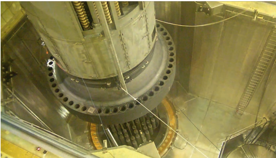
Fig. 21.3 RPV head lifting
