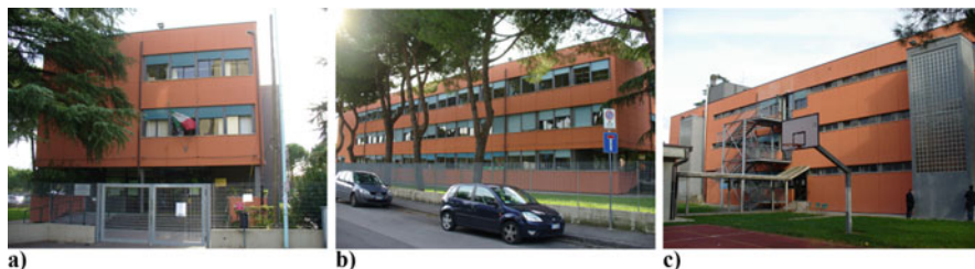
Fig. 18.2 School building: (a) frontal elevation where there are the portico and the entrance hall; (b) and (c) longitudinal elevations
