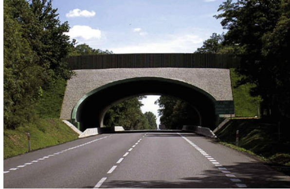
Fig. 3.1 Side view of soil-steel bridge
