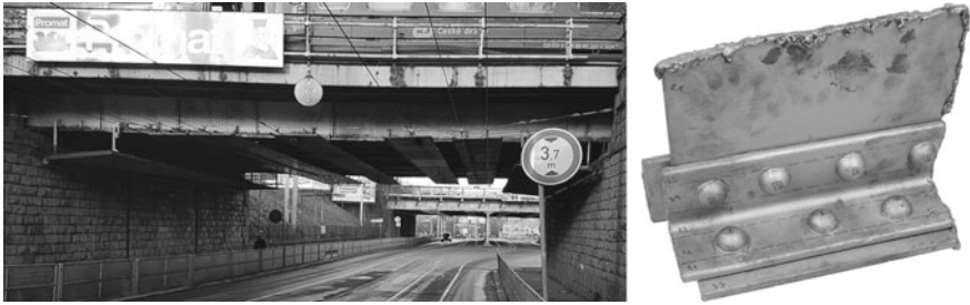
Fig. 1 Bridge before reconstruction [1]. Test sample—on the right
