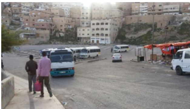
Fig. 18 The existing bus station (Source Researchers)
