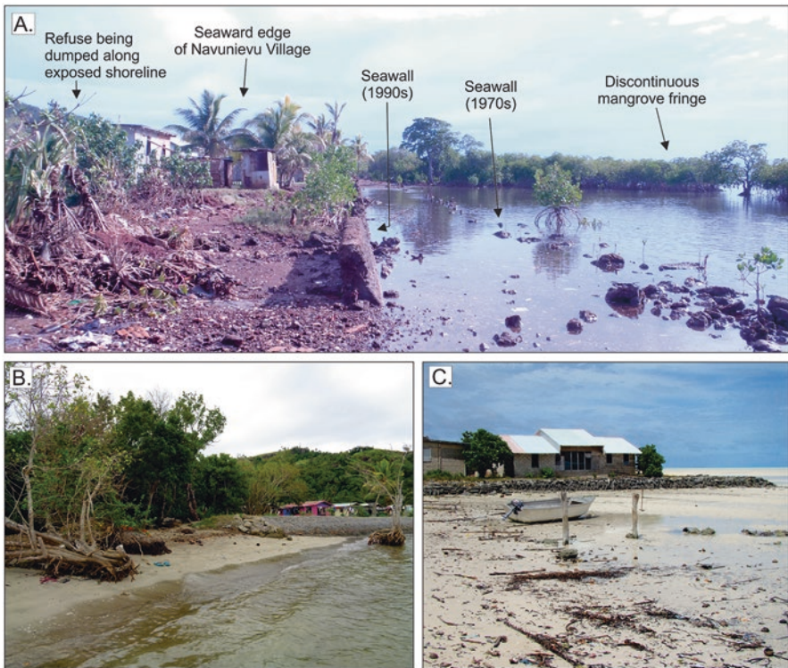
Fig. 14.1 Some issues with seawalls in rural Pacific Island communities. (a) Shows the coastline at Navunievu village (Vanua Levu, Fiji) where clearance of the mangrove fringe in the 1950s exposed the shore to wave erosion, to which local residents responded by building a (now-degraded) seawall in the 1970s and another (now crumbling) in the 1990s (photo by Patrick Nunn). (b) Shows the seawall, funded by USAID, along the front of Karoko village (Vanua Levu, Fiji) that does not extend beyond the village limits, places where shoreline erosion is visibly occurring (photo courtesy of Annah Piggott-McKellar). (c) Shows a house newly built on reclaimed land, bordered by a seawall made from uncemented reef rock, at Kabangani (Abemama, Kiribati). (Photo courtesy of Virginie Duvat)
