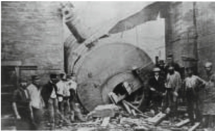
Fig. 1.2 Picture of boiler explosion due probably to caustic cracking
