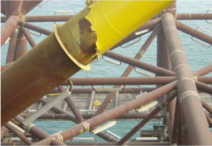
Fig. 1.23 Sacrificial anodes (the white handle-shaped objects protect the oil platform from corrosion. Image by Chetan, via Wikimedia Commons)
