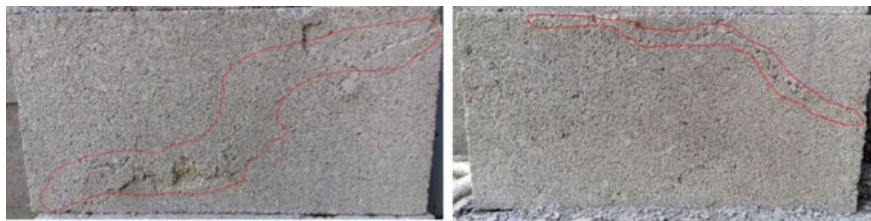
Fig. 11 Failure patterns of OPC hollow blocks
