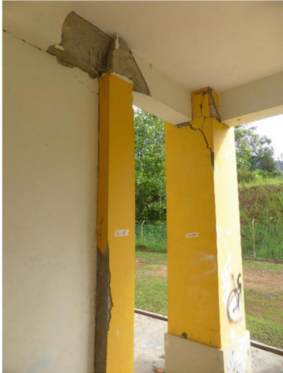
5th June 2015 earthquake in which significant damage was found mainly at column beam joints at first floor. Figure 14 shows damaged column beam joint of SMK Ranau building. In terms of seismic regulations, irregular condition such as a soft storey structure requires the application of special considerations in their structural design and analysis [3].
