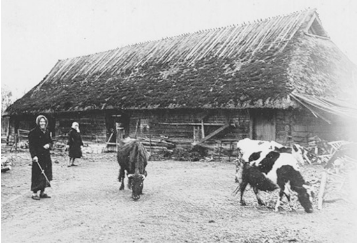
Fig. 15.2 Historical photograph of barn with cattle, Lümanda village, early twentieth century ( https://arhiiv.saartehaal.ee/2009/03/17/lumanda-muuseum-sai-naituse-tegemiseks-toetust/ )
