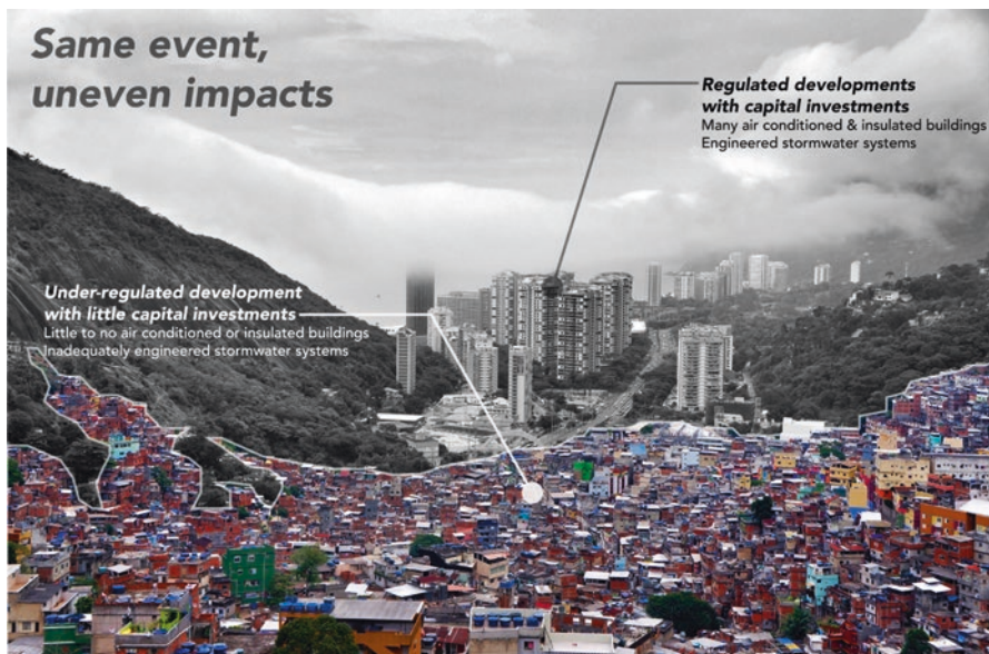
Fig. 17.2 The same meteorological event can result in uneven impacts for residents within adjacent neighborhoods because of differences in risk and vulnerabilities such as the quality of buildings and infrastructure. In urban systems, the impacts of extreme events are driven by how weather and climate interact with infrastructure, ecosystems and humans. (Source: Paul Coseo, YY, Brazil, 2012, https://yyinbrazil.wordpress.com/2012/12/01/yy-in-brazil-rio-de-janeiro-favela-rocinha-day-4/ )
