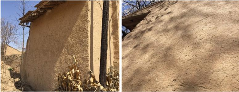
**Fig. 1.** Residential house built by the loess-PHW mixture: house wall (left-hand side) and enlargement of house wall (right-hand side)
