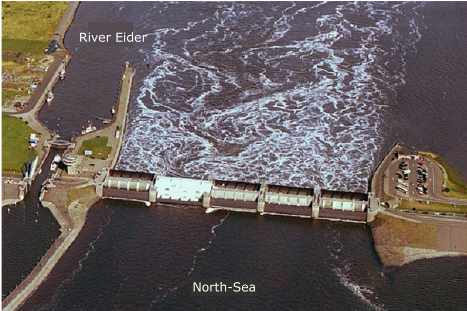
Fig. 1. Aerial photo of the “Eidersperrwerk” (source: WSA Tönning).
