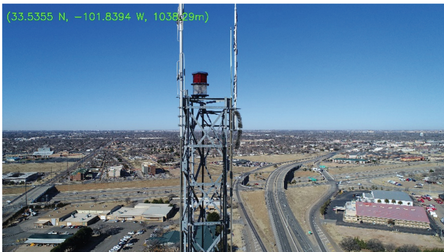
Fig. 5. Tower inspection with location coordinates overlaid on the image.
