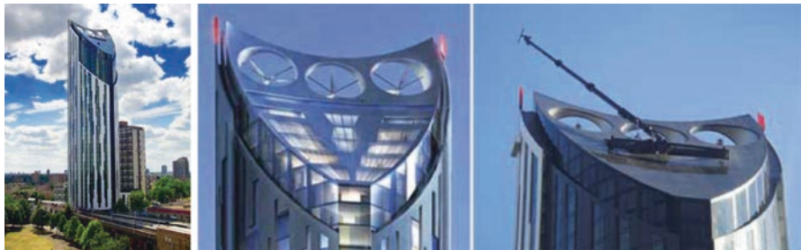
Fig. 30.14 The Strata SE1 residential tower in London [28]
