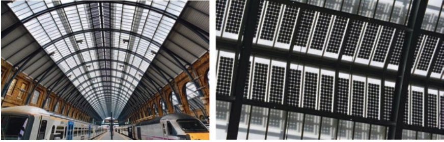
Fig. 30.5 St. Pancras King Cross Station BIPV system [18]
