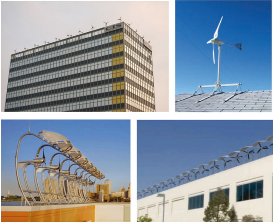
Fig. 30.11 Building mounted wind turbine with horizontal axis rotor [26]
