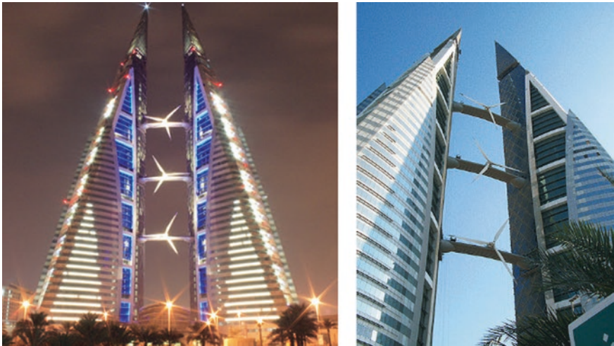
Fig. 30.16 Building augmented wind turbine, horizontal axis (World Trade Center, Bahrain) [26]
