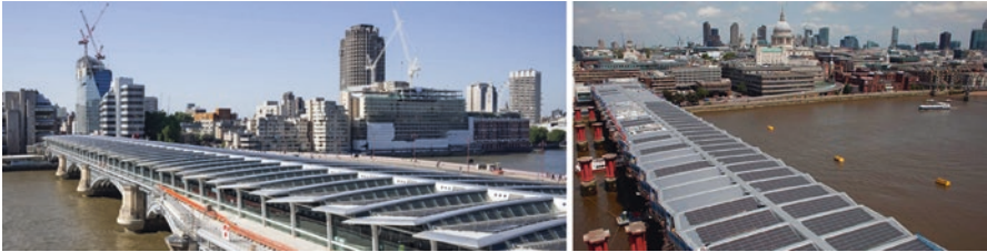
Fig. 30.6 Solar panels on Blackfriars bridge in London [19, 20]
