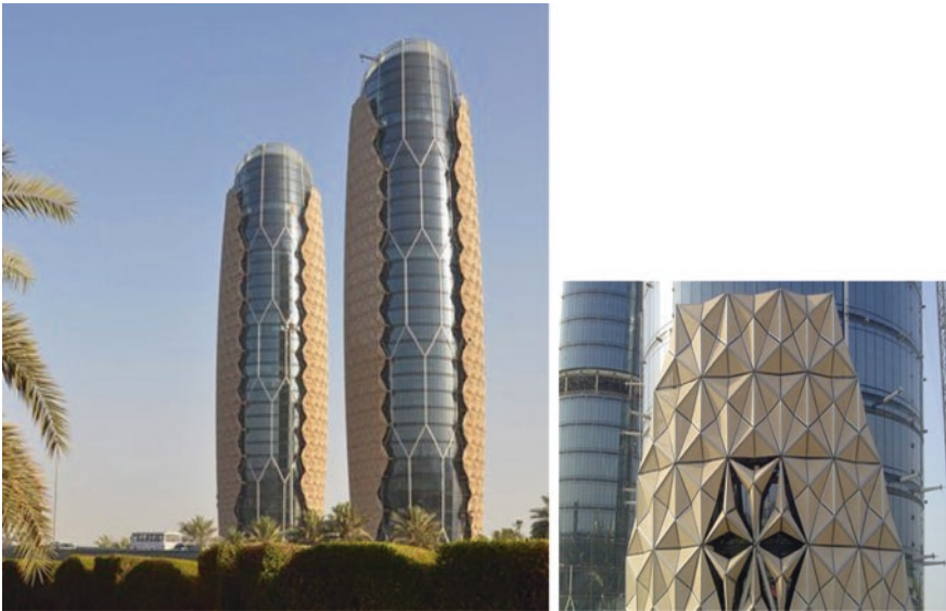
Fig. 29.17 The Green skyscrapers in Abu Dhabi, UAE
