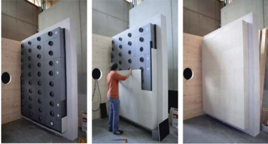
Fig. 23.22 Fast assembly time because dry construction site (no glue) [3]
