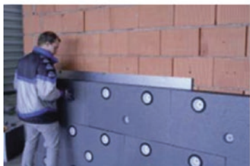
Fig. 23.25 Weather independent assembly tested winter -10\text{ }^{\circ}\text{C} [3]
