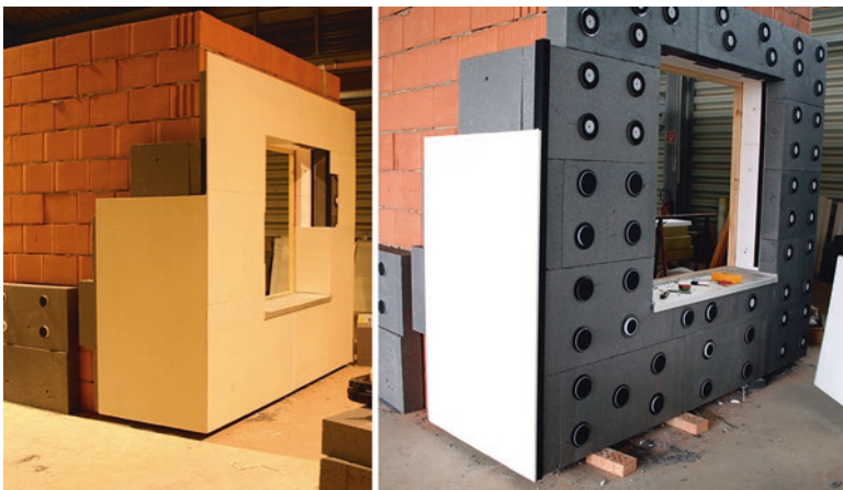
Fig. 23.13 Trial installations for conformability of craftsman [3]
