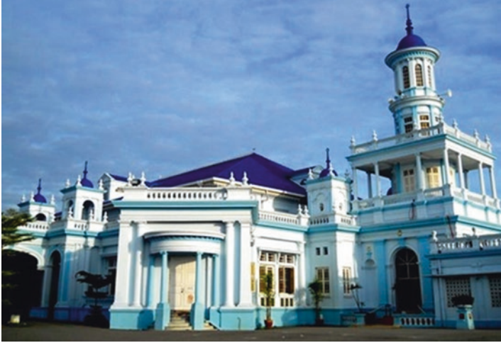
Fig. 18.11 Sultan Ibrahim Jamek Mosque
