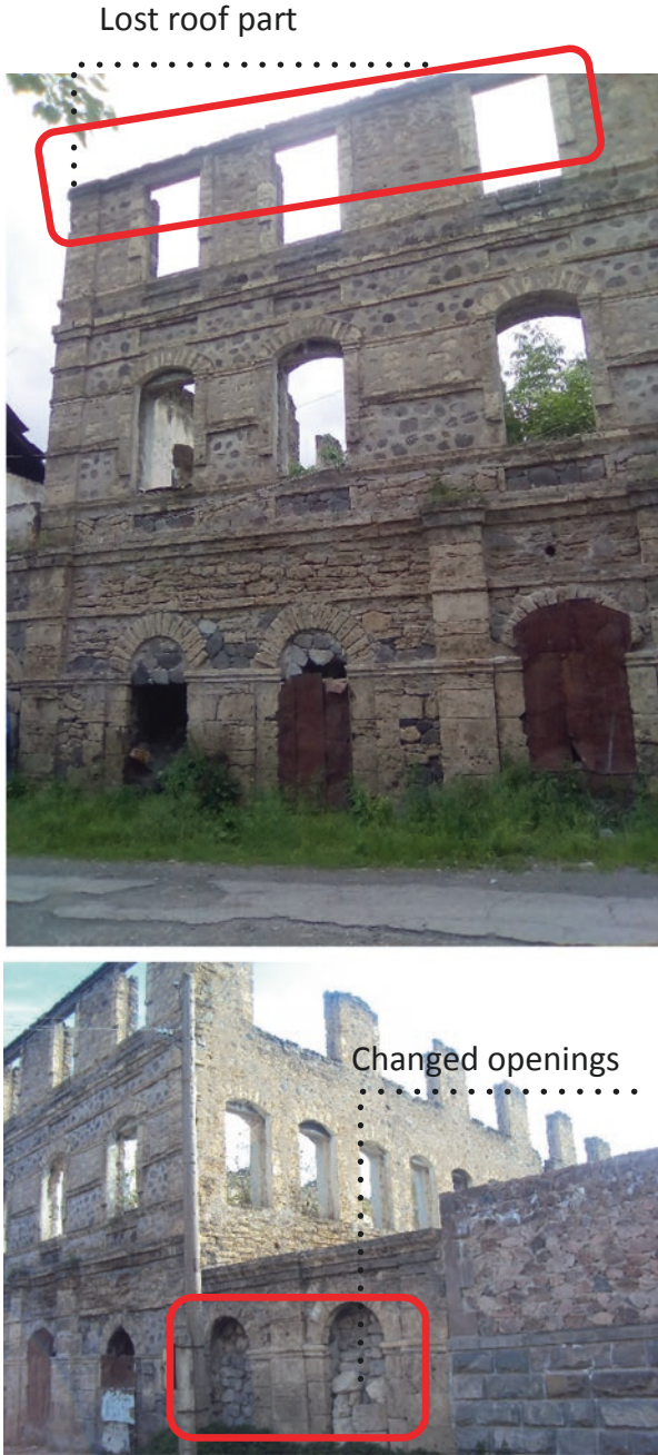
Fig. 1.3 Old bath building current condition
