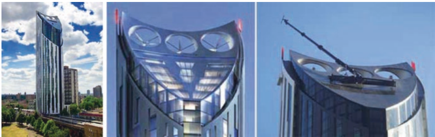
Fig. 30.14 The Strata SE1 residential tower in London [28]
