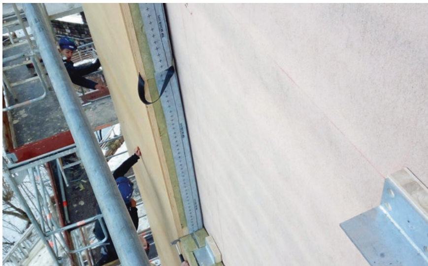
Fig. 22.11 Close-up of the junction elements between the façade and the EIF system. Source: https://www.agenziacasaclima.it/it/progetti-di-ricerca/sinfonia/sinfonia-risanamento-via-passeggiata-dei-castani-1783.html
