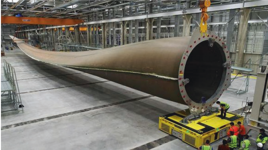
Fig. 43.4 A blade of the 12 MW Haliade-X wind turbine being built by GE
