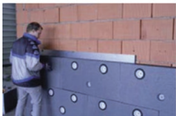
Fig. 23.25 Weather independent assembly tested winter -10\text{ }^{\circ}\text{C} [3]
