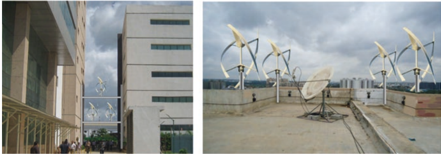
Fig. 30.13 Honeywell Orion Campus—India [27]
