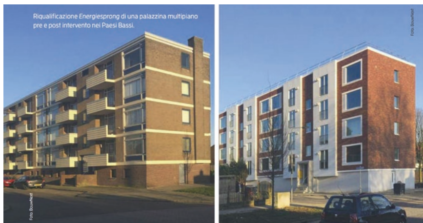
Fig. 22.3 Energiesprong requalification of a multistory building. Ante- and ex-post-intervention. Source: “Energiesprong Italia: un “salto energetico” per il retrofitting del futuro” edited by aZero in collaboration with Thomas Maiorin, aZero n. 24, pp. 48–57—EdicomEdizioni
