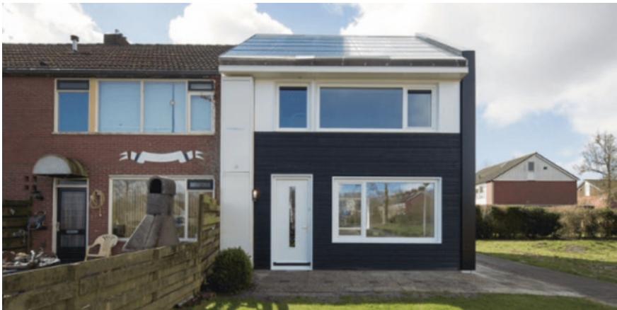
Fig. 22.1 Project by Ron van Erck for energy redevelopment with prefabricated panels. Source: Centomila case riqualificate in 10 giorni, a Rebuild il super-sistema dell'olandese van Erck—by Mila Fiordalisi, Edilizia e Territorio—Sole 24 ore, 25 June 2015
