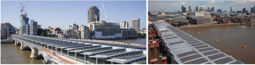
Fig. 30.6 Solar panels on Blackfriars bridge in London [19, 20]
