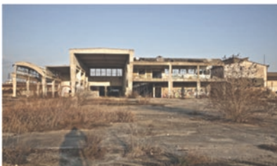
c. Abandoned of site and building
