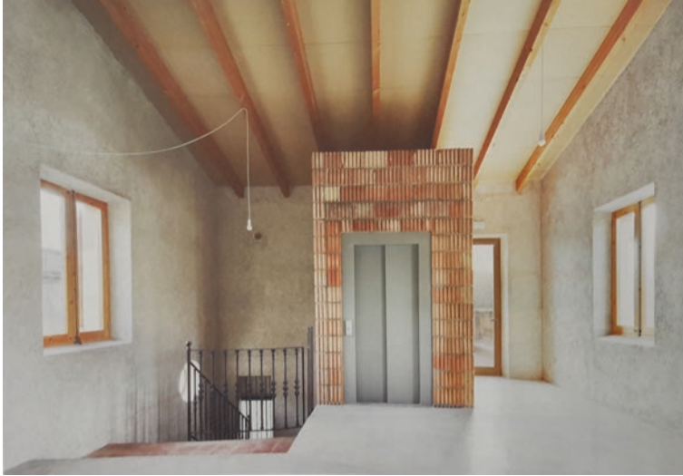
Fig. 19.11 Mallorca winery refurbishment using cork and ceramic blocks
