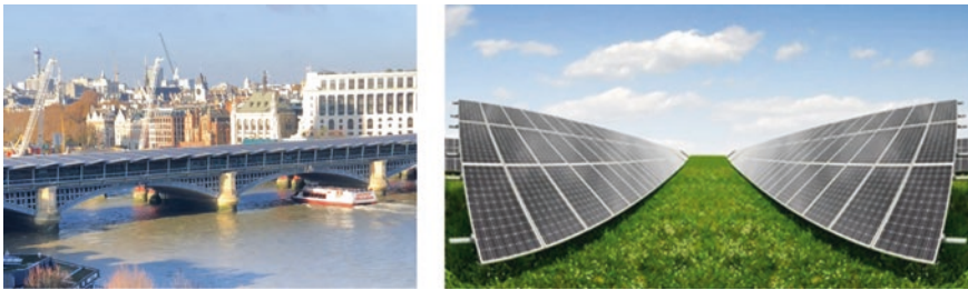
Fig. 27.8 Blackfriars Bridge 5 MW, London and solar farm near Reading
