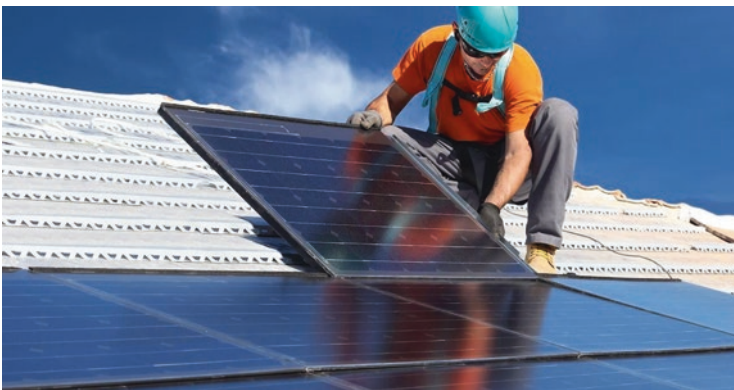
Fig. 29.18 Fixing solar panels on the roof of the houses
