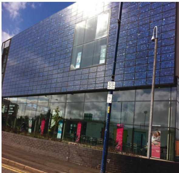
Fig. 30.1 BIPV system powering Manchester College of Arts and Technology's library
