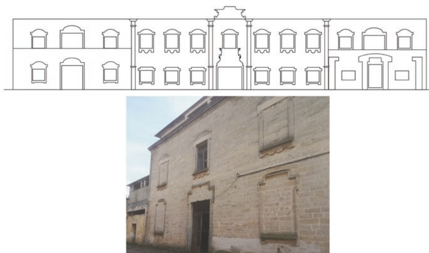
Fig. 19.2 Façade in Lecce stone with framed windows and doors; drawing (top) and picture (down)
