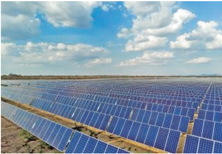
Fig. 27.10 300 MW PV farm installed in Brazil in 2019 at a cost of US$ 300
