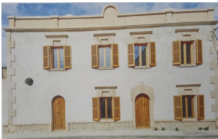
Fig. 19.10 Main façade of the Mallorca winery [4]
