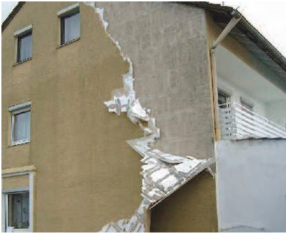
Fig. 23.2 Demolition of EIFS (Source: https://www.immoclick24.de/wp-content/uploads/2015/07/MM05-13_2_500x400.jpg )
