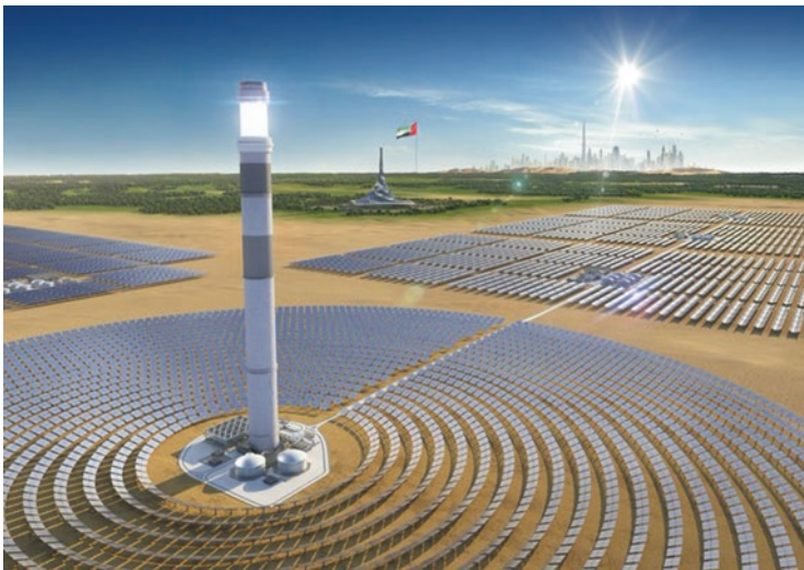
Fig. 29.20 World's biggest Concentrated Solar Power project in Dubai
