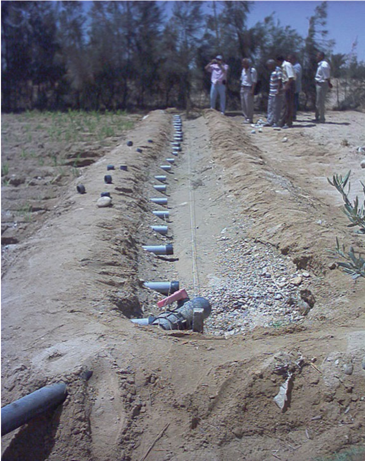
Fig. 10 After installation and evaluated of spill pipes with excavated channel
