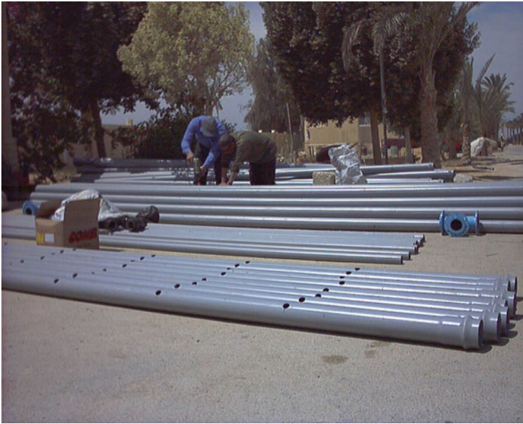
Fig. 13 Preparation and collection of controlled perforated pipes (CPP)
